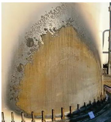
will seep in to the fracture, and corrosion will begin. Damage can occur for a multitude of reasons during transportation and erection of the towers, and often requires in-field repair. Ideally, the standards maintained by the National Association of Coatings Engineers (NACE) and the Society for Protective Coatings
